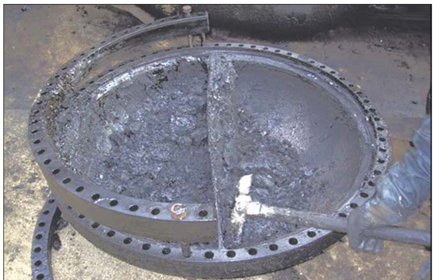
Figure 6 Manual removal of coke formation in the S&T turning chambers in a high-fouling visbreaking process
