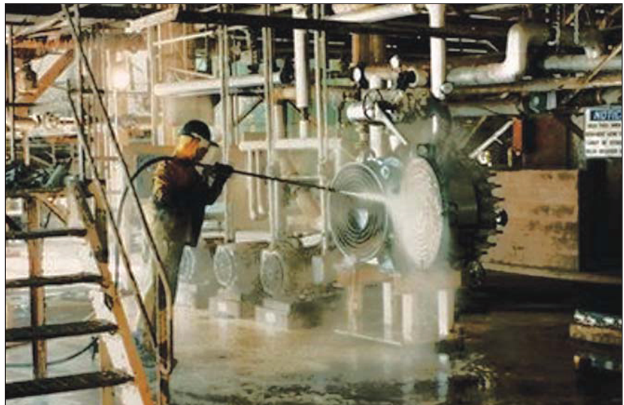
Figure 4 High-pressure water jet cleaning of the SHE heat-transfer surface
